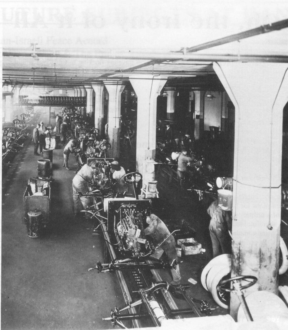
Driving down the line: Model T chassis assembly line in Detroit (1914). [Ford of Canada Archives]
